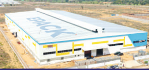
Unit 3 Ghiloth, Rajasthan
