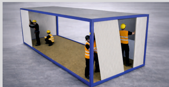
WALL PANEL INSTALLATION
