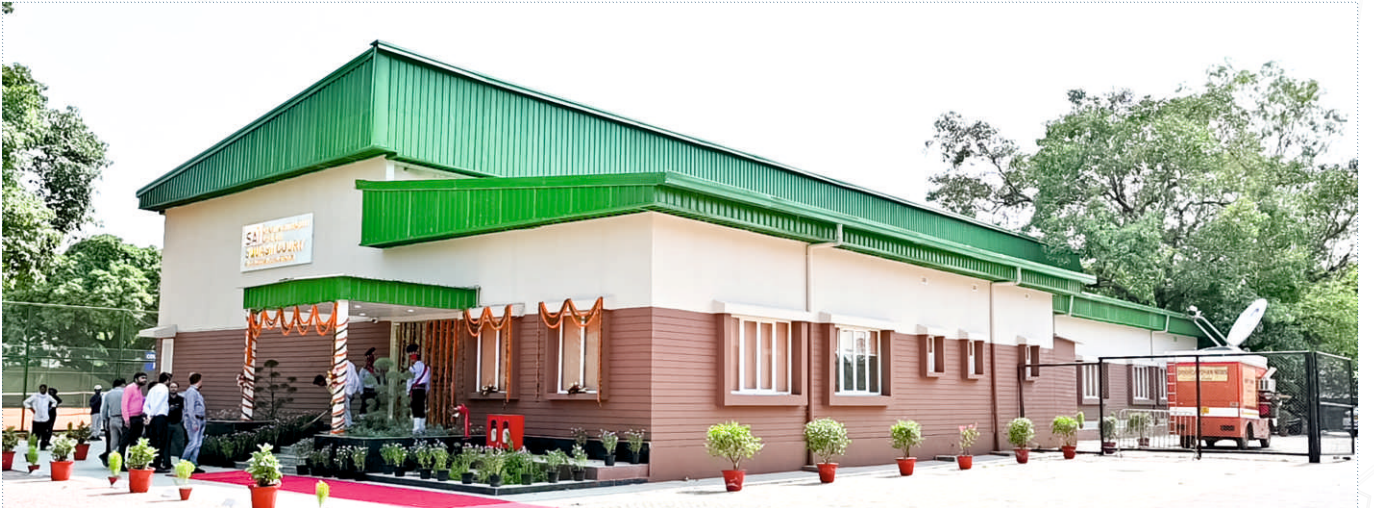
LGSF Squash Court Building For SAI
