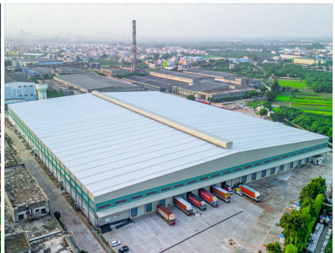
Warehouse Building For Pallika Town
