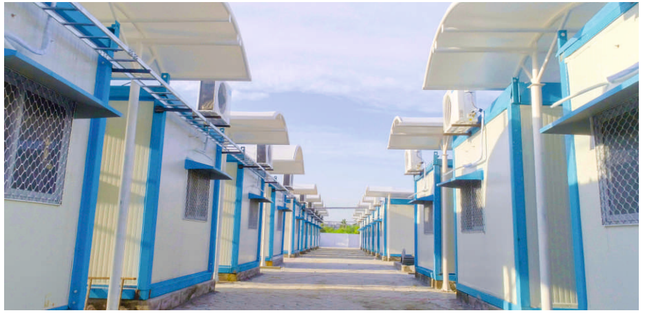
Temporary Staff Accommodation
