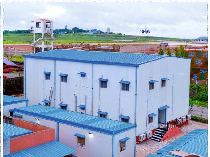
Site Infrastructure For Airports Authority of India
