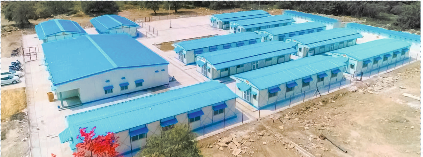
Prefabricated Site Infrastructure For Chambal Fertilizers
