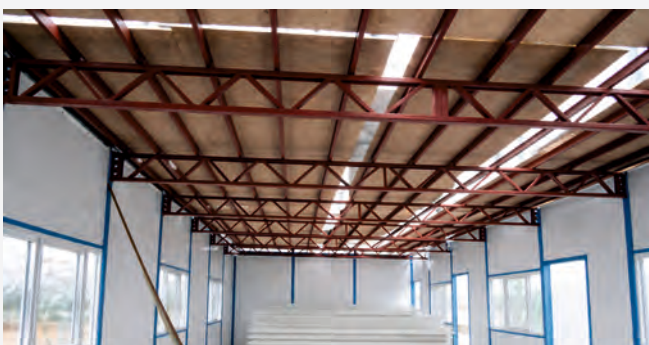
FLOOR JOIST & PURLINS
