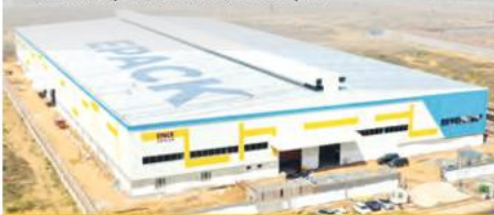
Unit 3 Ghiloth, Rajasthan
