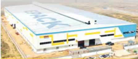
Unit 3 Ghiloth, Rajasthan
