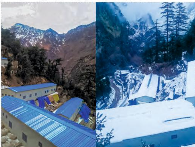
Hydro Project Site Infrastructure For JP Associates
