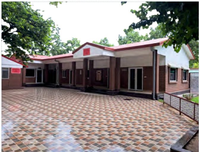
Army Accommodation At Kashmir House For MES
