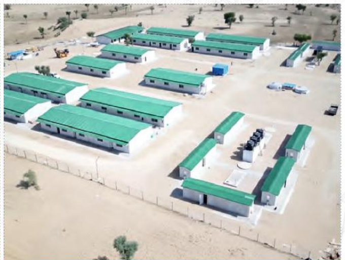
Worker Accommodations For Sunbreeze
