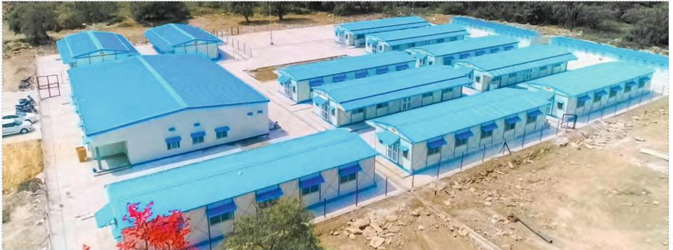
Prefabricated Site Infrastructure For Chambal Fertilizers
