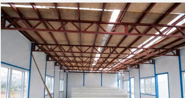
FLOOR JOIST & PURLINS
