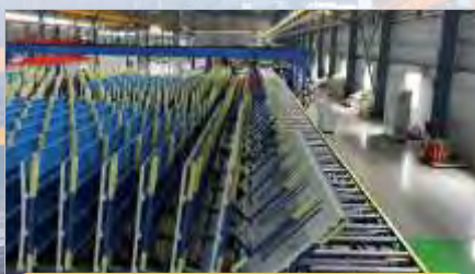
PANEL COOLING MACHINE
