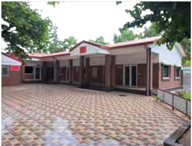
Army Accommodation At Kashmir House For MES
