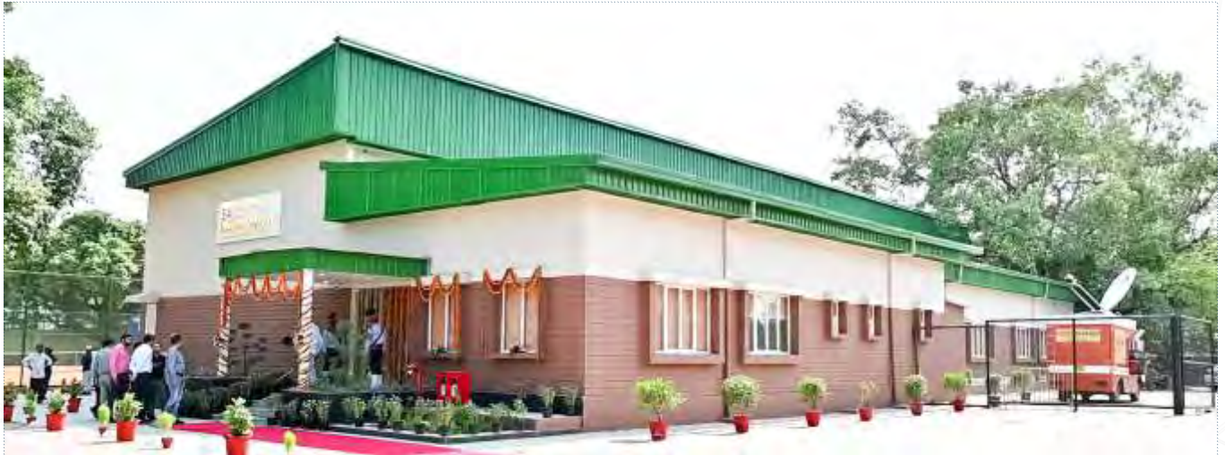
LGSF Squash Court Building For SAI
