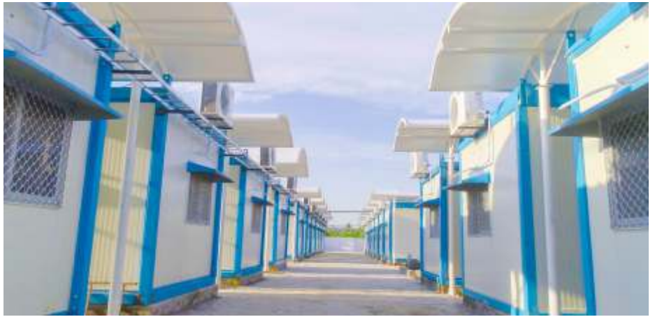
Temporary Staff Accommodation
