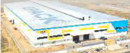
Unit 3 Ghiloth, Rajasthan
